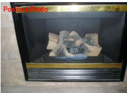
Photo: 2. Gas fireplace working. (1)
