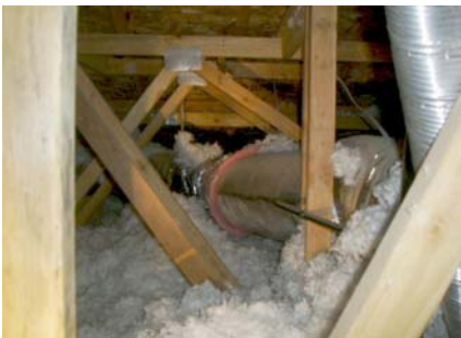
Photo: 9. View of attic. (1)
